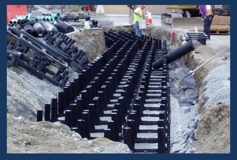
A network of frames (each with six rigid vertical posts) is positioned on the base material and anchored in place. These frames can be stacked one, two, or three high allowing for varying capacity.
