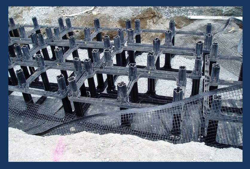
"Strongbacks" are placed on top of frames. They are only required during installation and compaction of soil to help hold frames in place.
