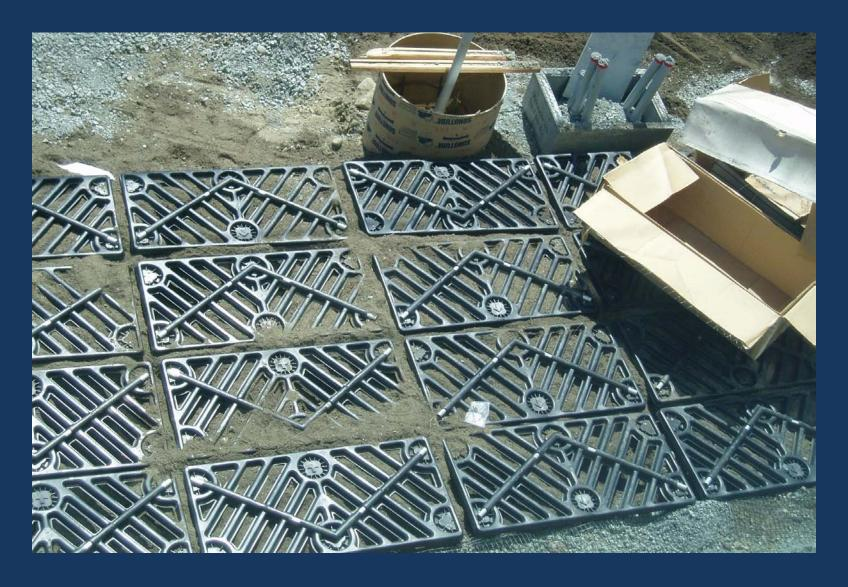
The deck is a rigid platform with ample openings for air and water penetration. Two diagonal channels house galvanized steel tubes to help prevent deformation.
