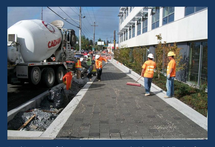
For this portion of the project, pavers spaced with gravel (allowing for infiltration) are placed over the newly installed root box system for a public sidewalk. Trees will be planted soon.
