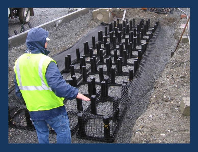
Geogrid is placed around the entire system to properly hold soil in place.
